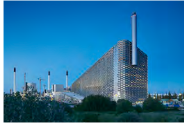
AMAGER BAKKE / COPENHILL
