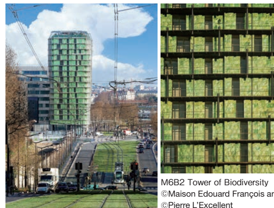
©Atelier Tsuyoshi Tane Architects
