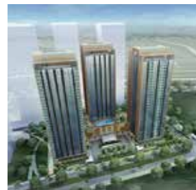
Project in Indonesia
