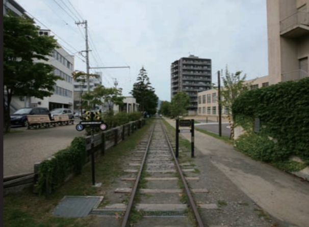
鉄道跡 Former Line
