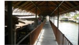
2b Railed pedestrian walkway B
